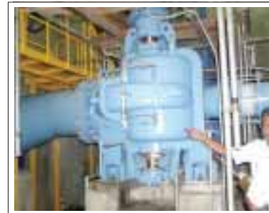
Ambatale water transmission pump: 45m 3 /min x 850kW x 2units
