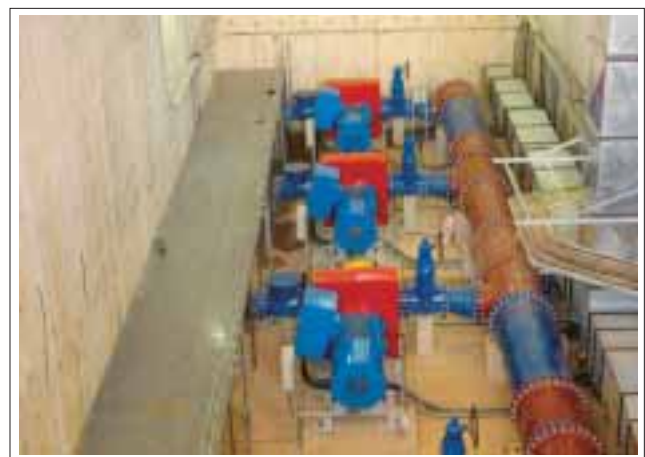
High Lift Pump
