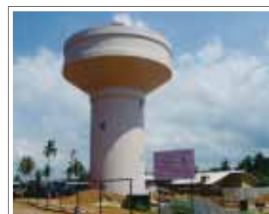
Kandana elevated water tower: V.1000m 3 x H.25m
