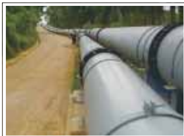
Church Hill gravity water transmission main Dia. 1000mm SP & drain water pipe Dia. 600mm SP
