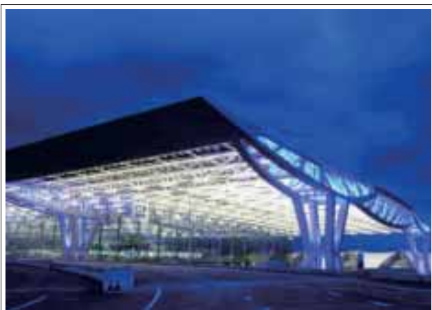
" Supertruss " at Main Terminal spans 100 m supporting the world ' s largest single roof
