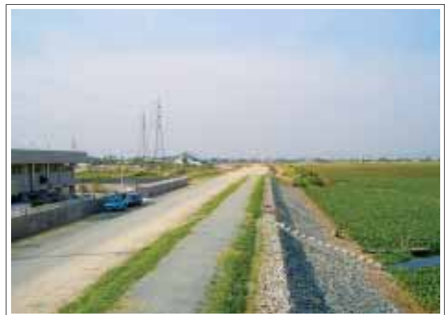
Completed Dike and Pumping Station
