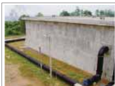
Church Hill ground reservoir: RC: L.66m x W.33m x H.9m - V.18000m 3
